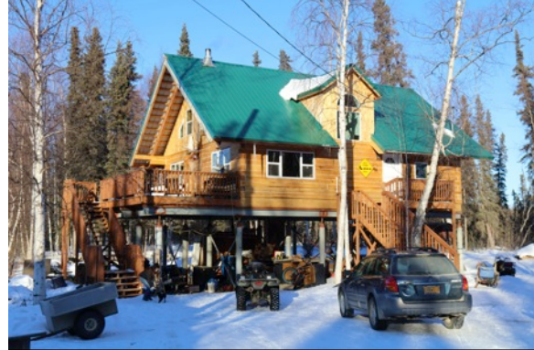
The mayor's house in Galena. As in Edeytsy, stilts are one answer to the flood problem.
