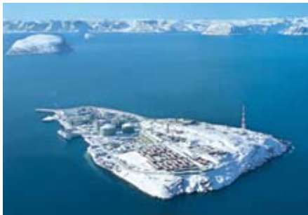
Oil extraction, Melkøya plant, Snøhvit field, near Hammerfest, Norway | Photo by Eiliv Leren, Statoil ASA
